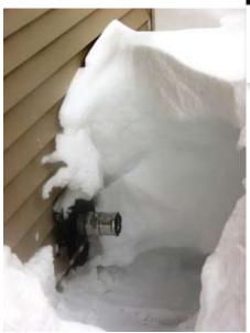
vents can affect the combustion process, which can create carbon monoxide, which could possibly enter the home through nearby openings.
